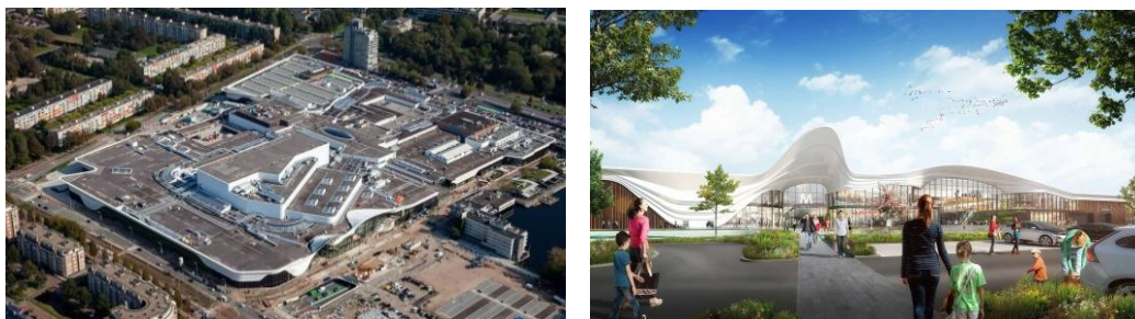
Gambar 1. Eksisting Westfield Mall Of The Netherlands
